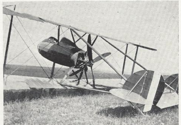
Pemberton-Billing single-seater pusher Scout with 50 h.p. Gnome engine
