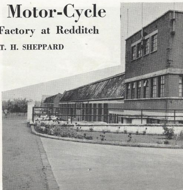
The small Redditch factory, part of which is concerned with the manufacture of the Sunbeam motor-cycle
